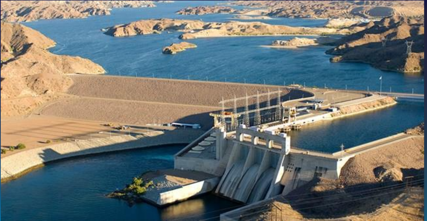
Davis Dam, Nevada
